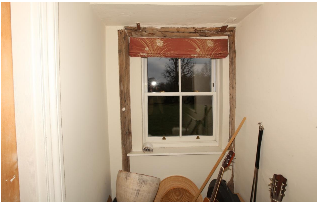
Illus. 28. The gallery terminates at a doorway with broad chamfers to its jambs and lintel that terminate well above the ground in the manner of the early-17 th century. The fabric is hidden elsewhere in this south-eastern gable but it appears to consist of rendered early brickwork as noted in illustrations 3-5. This doorway presumably opened into a missing brick wing at the end of the gallery that was probably added when the building was converted into a house for a member of the Poley family.
