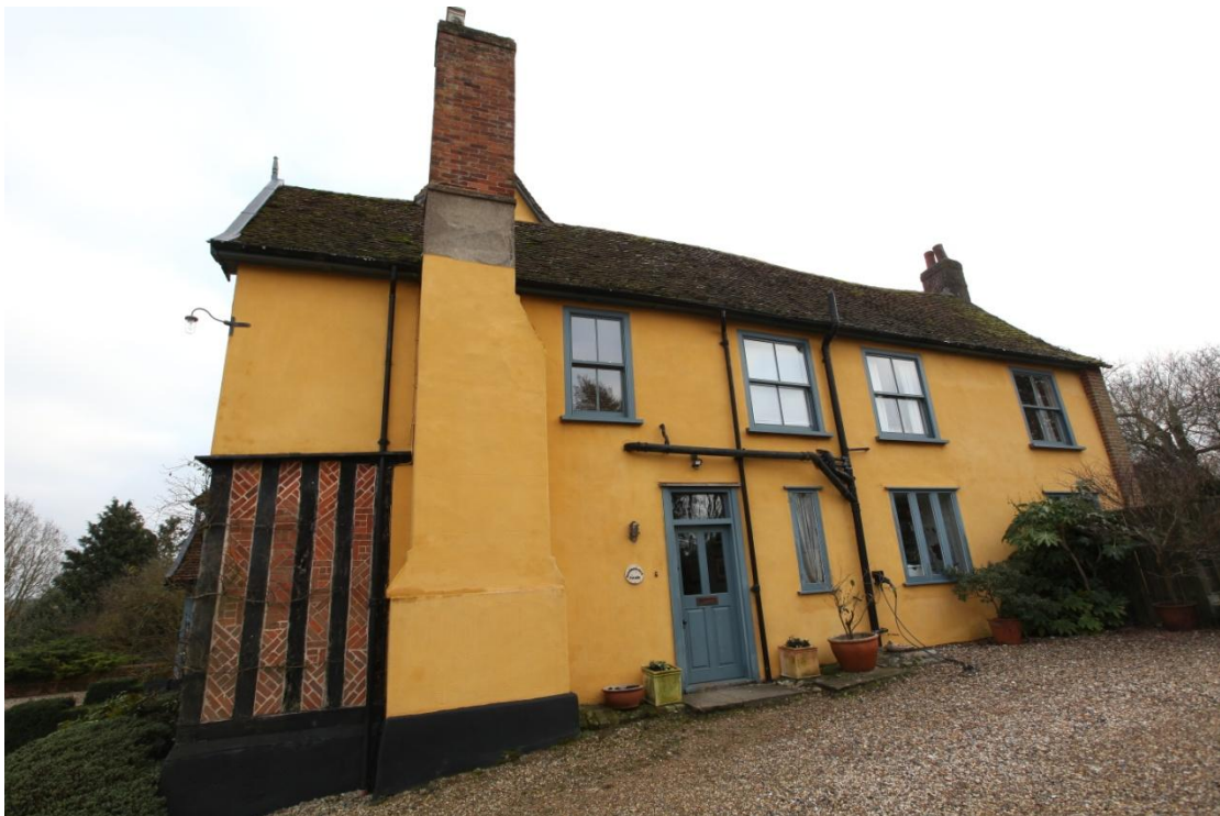
Illus. 6. The north-western side wall of the late-15 th century five-bay parlour cross-wing, which retains its original crown-post roof throughout. The wing is highly likely to have been jettied to its north-eastern facade on the left, but any such feature has been cut off rather than under-built. The present corner post dates from the late-Victorian refurbishment, as does the brick nogging and most but not all the studwork to the left of the ostensibly 19 th century chimney.
