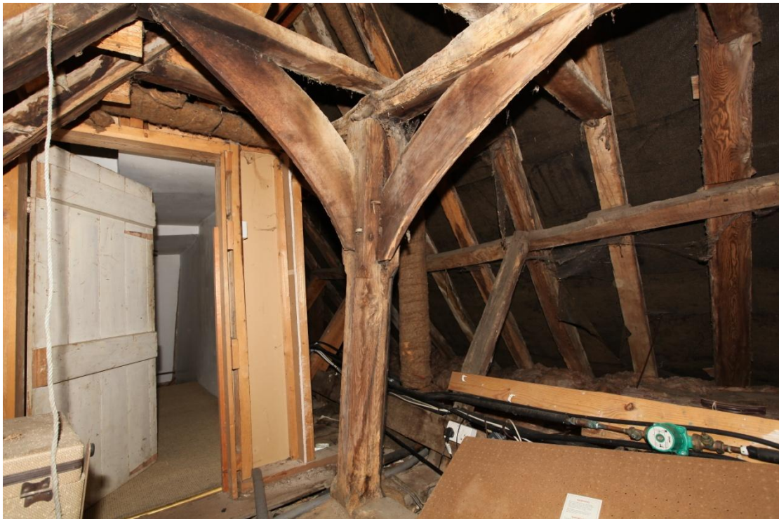
Illus. 18. The neatly chamfered crown post of the front parlour chamber, above the ogee-moulded ceiling in illustration 7. The chamfers are broach-stopped at the bottom and step-stopped at the top. The roof timbers are smoke-stained due to leakage from the open hall and the once jettied front (north-eastern) gable has been truncated and rebuilt as there are no mortices for collar braces in either the purlin or its central stud.
