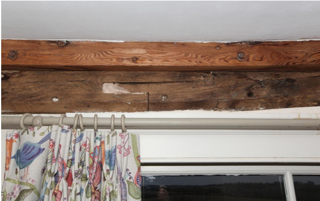
Illus. 33. A detail of the unusual scarf joint in the north-eastern roof-plate in illustration 32, which appears to be edge-halved and bladed rather than face-halved in the usual manner of the late-16 th and early-17 th centuries. It indicates a transitional date in the mid- to late-16 th century when traditional edge-halved and bridled joints were becoming outmoded.
