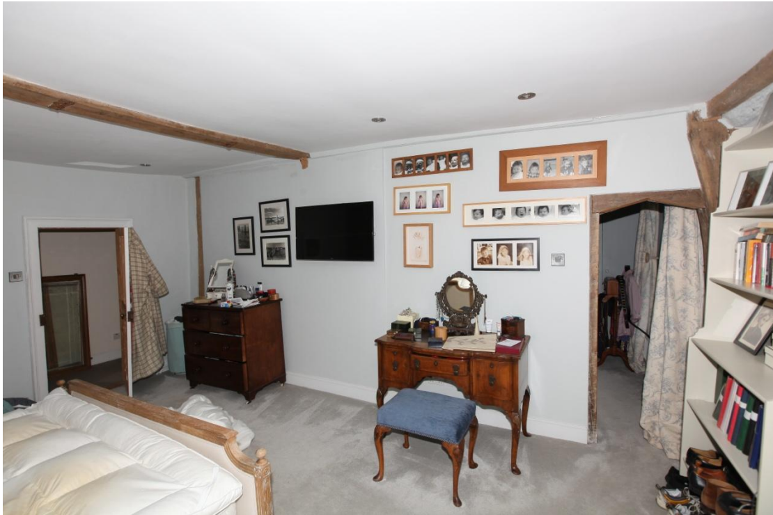
Illus. 37. The south-eastern wall of the bedroom above the sitting room, showing an inserted door arch to the right of the present chimney which is hidden by render at this level.
