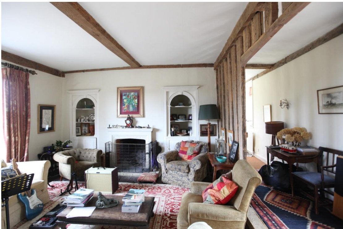
Illus. 22. The modern sitting room in the 16 th century range looking south-east towards its 20 th century fireplace with the jettied gallery on the right. Pegs for vertical studs are visible in the binding joist above the 18 th century-style shelf unit to the left but their absence elsewhere indicates a chimney always occupied this position (but faced south-east as this room was heated by a missing chimney in the foreground).
