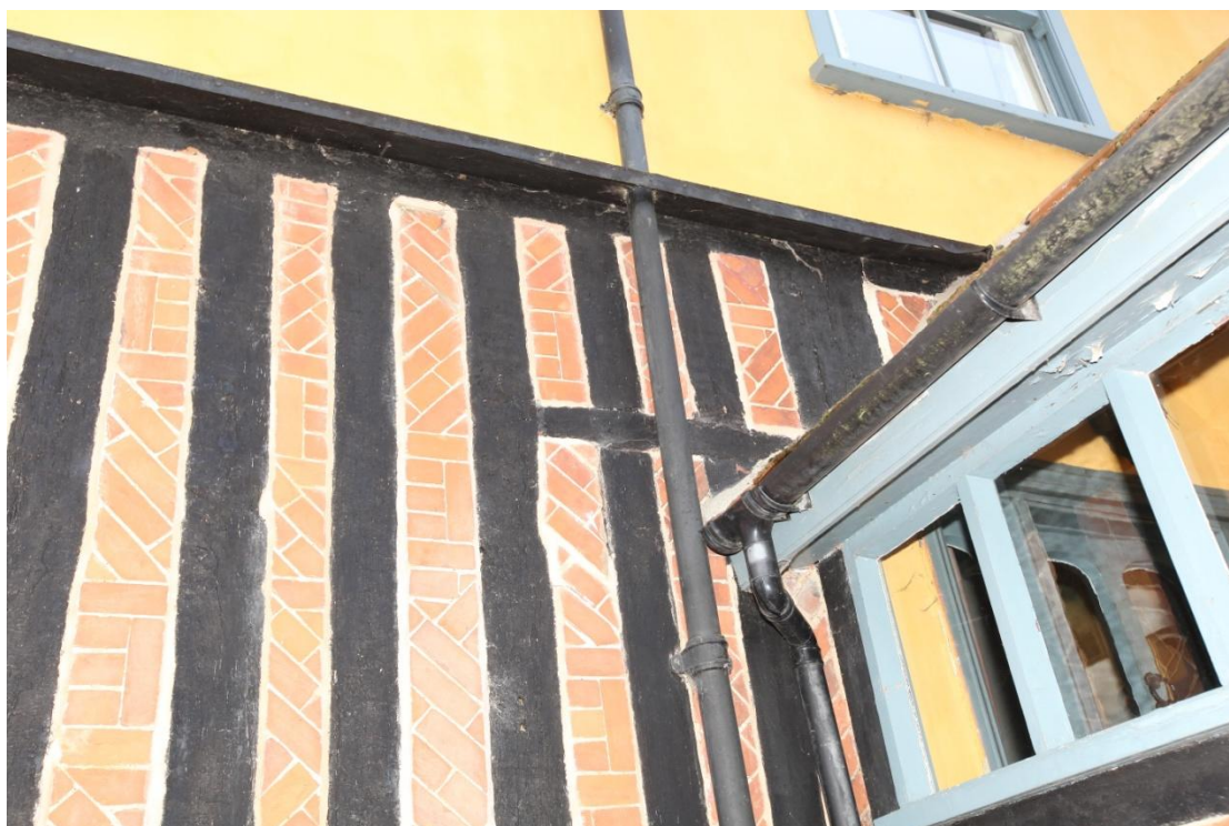
Illus. 2. A detail of the facade in illustration 1 showing the pegged lintel of an original ground-floor door that was matched by another on the first floor immediately above. These doors would have opened either into an entrance porch with a first-floor chamber or a turret containing a stair or privies. The brick infill dates only from the Mock Gothic remodelling but replicates the original nogging (illustration 27).
