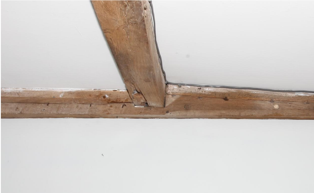
Illus. 35. A detail of the tie-beam in illustration 34 showing the end of its stud pegs and chamfer with a gap to the left that corresponds with the apparent chimney aperture on the ground floor. The ground-floor binding joist beneath lacks a chamfer where it abutted the missing brickwork in the same way.
