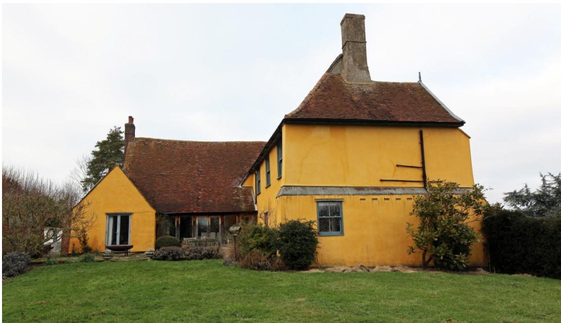
Illus. 4. The house from the south-east showing the rendered brickwork of the gable with the 20 th century glazed lean-to dining area against the parlour wing in the rear. The ground-floor gable window occupies the position of a late-16 th or early-17 th century doorway with chamfered jambs at the end of the gallery, suggesting it opened into a missing structure in the foreground of which the brickwork presumably forms a part. More evidence of the building's arrangement is likely to be revealed if the render is ever renewed.
