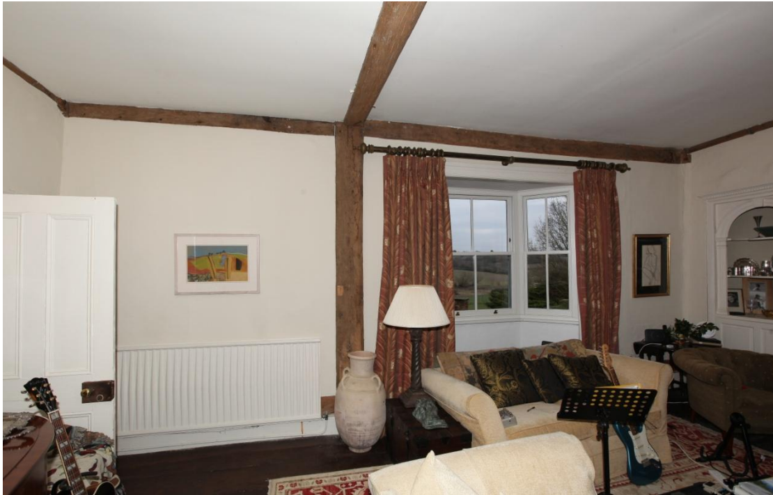
Illus. 23. The front (north-eastern) wall of the sitting room, with the position of the blocked door visible externally on the left (illustration 2). The exposed mid-rail of the internal wall against the present stair lobby to the extreme left contains an uninterrupted series of pegs for a solid wall, and the position of any door is unclear. A wide gap in the stud pegs in both the upper and lower edges of the mid-rail above the present window indicate a large original bay window, probably of brick, that extended to the upper storey.
