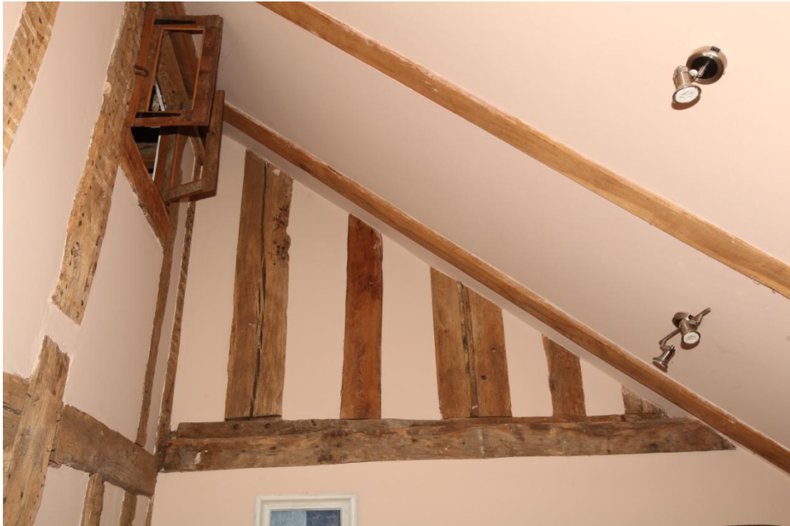
Illus. 13. The small exposed section of 16 th century jetty bressumer in illustration 11, overlapping the narrow stair bay of the earlier parlour wing on the left. The bressumer is largely concealed by a later horizontal timber, but the twin pegs of the Tudor range's corner post are clearly visible. The equivalent of this timber in the opposite wall is shown in illustration 32 and forms a single storey-post rising from the ground sill.
