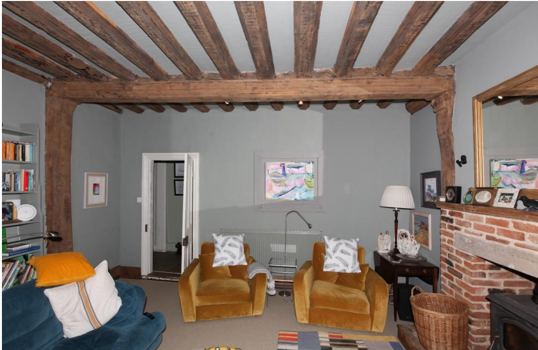
Illus. 7. The two-bay front parlour as seen from its north-eastern facade. The fireplace in the external chimney shown in illustration 6 on the right is modern. This room initially extended to the south-western wall of the present entrance passage, which is visible through the open door in the rear. This passage aligns with the Tudor gallery and may represent a contemporary insertion.
