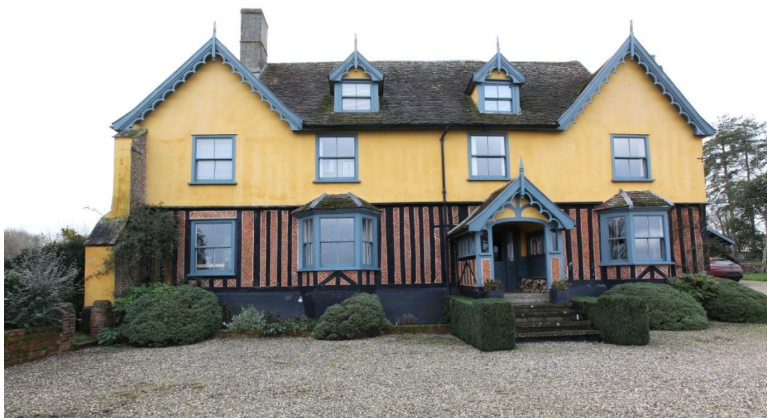
Illus. 1. The north-eastern facade of the house, with the late-medieval parlour crossing on the right and the highly unusual late-16 th century range on the left. The false matching gable to the extreme left was probably added as part of a late-19 th century Mock Gothic refurbishment that included the porch. Some of the exposed framing survives from the 16 th century and the ghosts of internally hidden, closely-spaced studs can be seen through the first-floor render.
