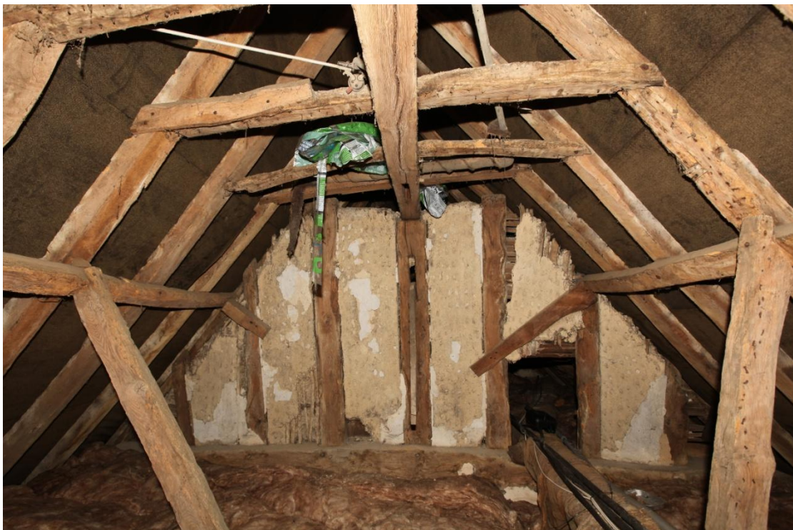
Illus. 20. The roof of the single-bay central parlour chamber showing its original crown-post structure with inserted through-purlins supported by raking struts. The original brace survives but has fallen out of its mortice in the collar purlin and is suspended by a peg from the crown stud. Fragments of original lime plaster adhere to the wattle-and-daub. This space was formerly open to the first-floor room beneath.
