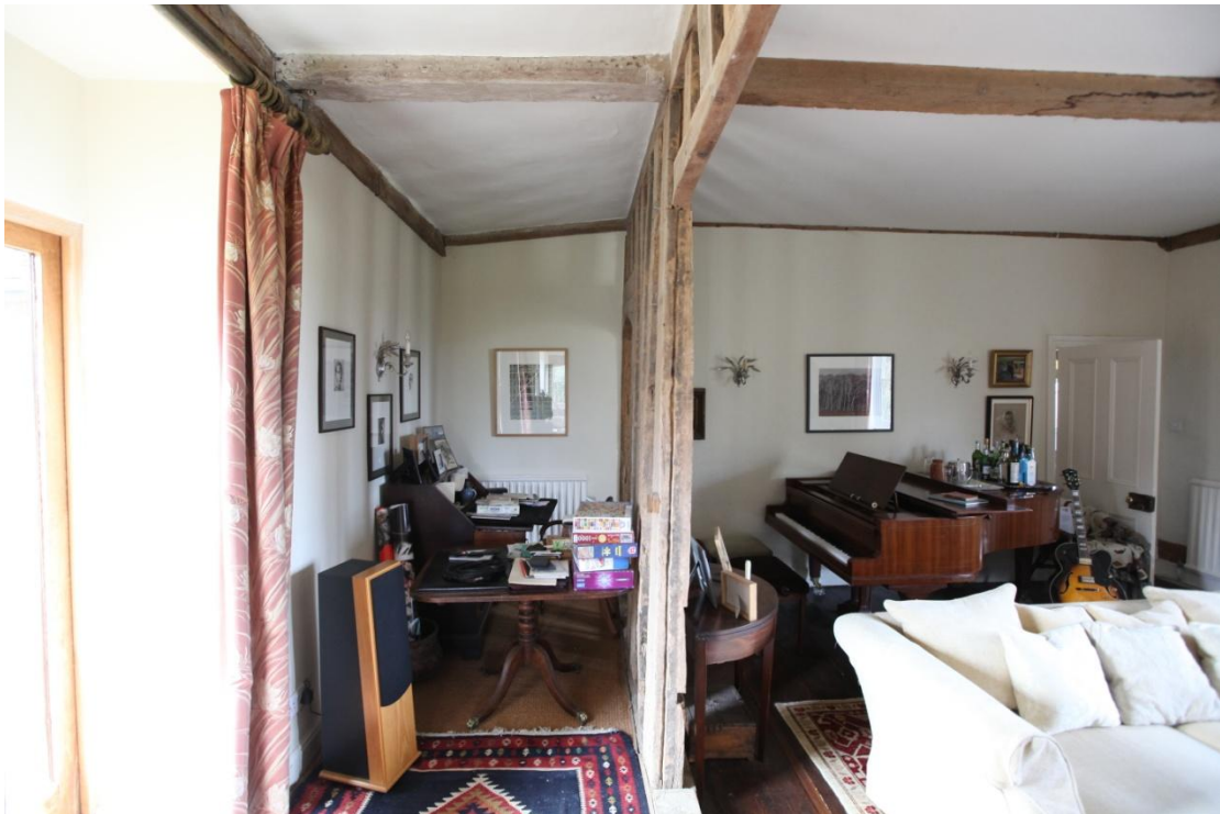
Illus. 30. The gallery from the south-east, showing the thickness of the apparently brick wall that replaced the jetty on the left. The exposed inner jetty plate contains pegs for a seemingly solid wall opposite the arched door in the rear, but in fact almost certainly for a section of framing above a matching external door. Wide gaps in the mortice pegs elsewhere in this plate indicate the presence of arches or balusters. The underside of the plate may retain rebates or mortices for these features, and it is possible that some original elements of the missing wall were re-used in the later fabric.
