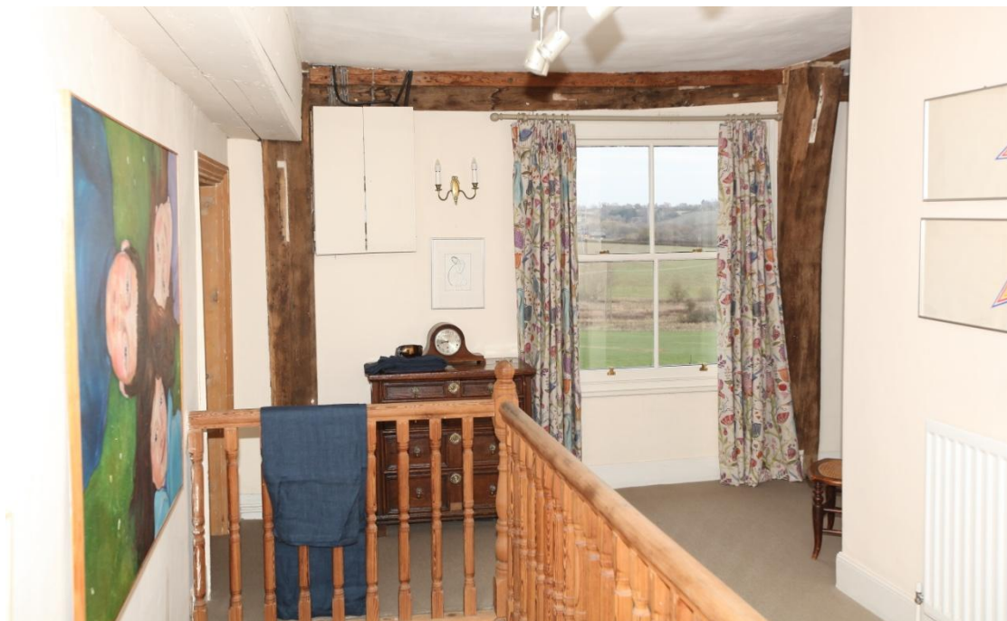
Illus. 32. The first-floor landing of the late-19 th century main staircase, showing the latter's stripped pine balustrade and handrail in the foreground. The framing of the cross-wing on the left is hidden by plaster, but the corner post of the 16 th century range contains an empty mortice for an arch-brace to its tie-beam demonstrating that the later structure was open-framed against the earlier.
