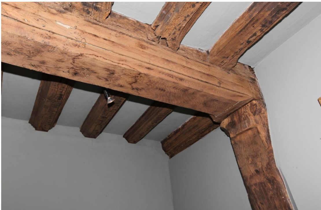
Illus. 8. A detail of the front parlour ceiling in illustration 7 showing its ogee-moulded principal and common joists, with the former supported by a shaped corbel block on the storey post. The joints are simple soffit tenons. Mouldings of this form are typical of the late-15 th and early-16 th centuries, and are common in local towns such as Lavenham, but at 2.75 m or 9 ft the impressive height of the ceiling indicates exceptional status.
