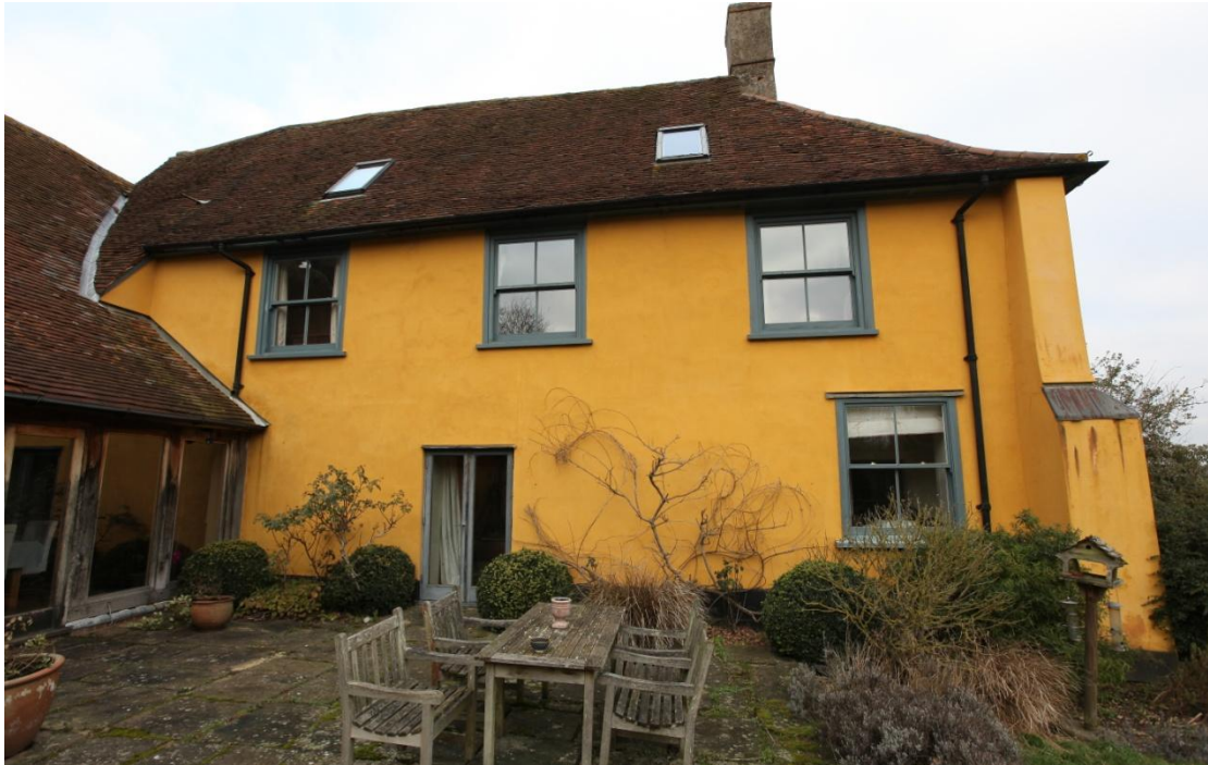
Illus. 5. The render of the south-western wall conceals a jettied upper storey that originally projected from a ground-floor wall that formed an open arcade or balustrade against the internal gallery in illustrations 29-30. The jetty appears to have been under-built in brick, but the lower wall may include some repositioned original timbers.
